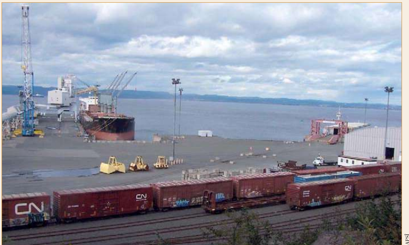
View of operations at La Relance Terminal of the Port of Sept-Îles which registered a traffic increase in 2008.
