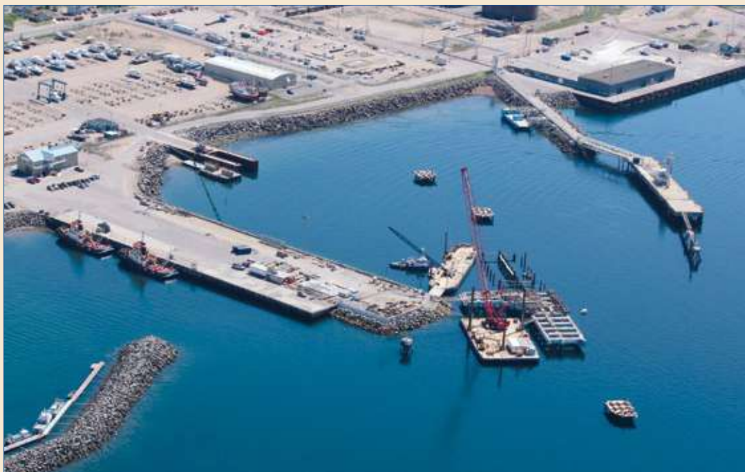
Future of the Port of Sept-Îles looks bright in light of promising development of the iron ore sector.
