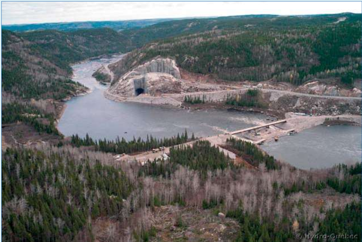
Aerial view of construction work well in progress at the gigantic La Romaine hydroelectric project.
