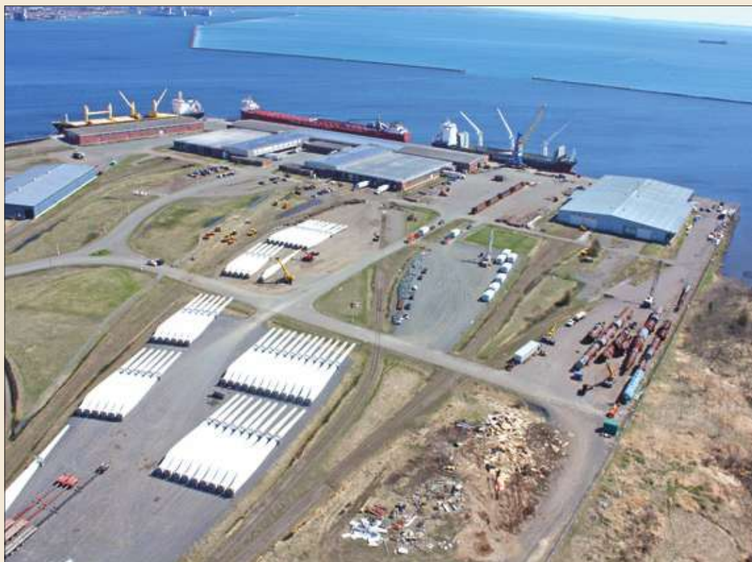
The Port of Thunder Bay at the tip of Lake Superior is continuing to show brisk volumes in grain and has also been handling a wide variety of general and project cargoes, including wind turbine components from Brazil for a wind farm near Wawa, Ontario.
