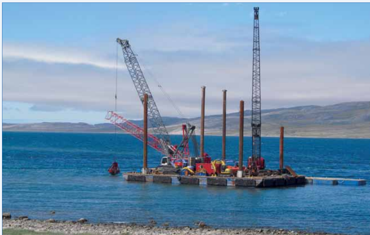
Rental of Ocean maritime equipment to an entrepreneur for the construction of a deepwater quay in Nunavik, northern Québec.
