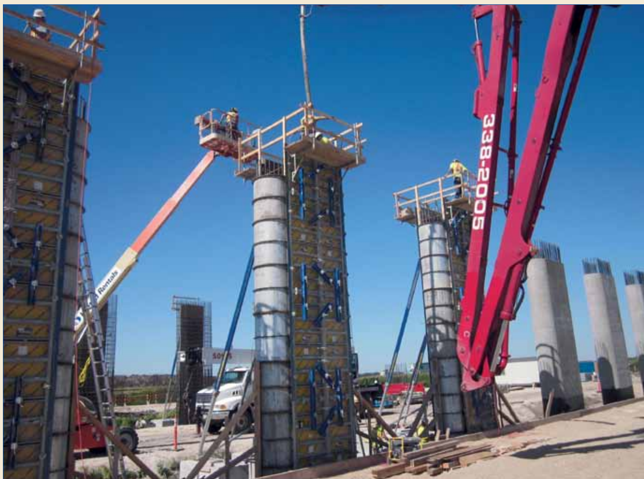
The development of CentrePort Canada Way, Manitoba's inland port, includes the construction of a $212.4 million divided expressway.
