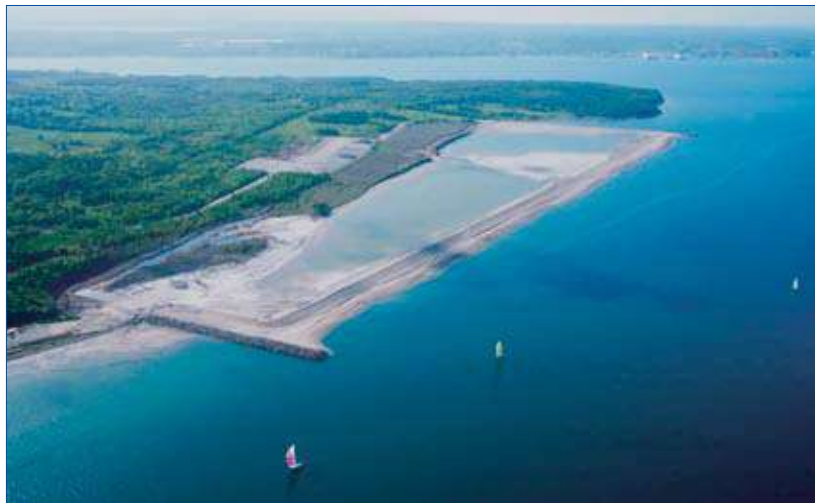
Aerial view of the greenfield site at Sydney Port proposed for a one million TEU container terminal.
