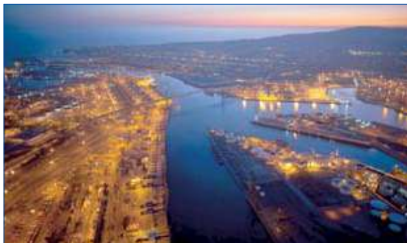
The Los Angeles Harbour Commission recently approved $7.5 million for the final phase of a main channel deepening to a 53-ft depth.
