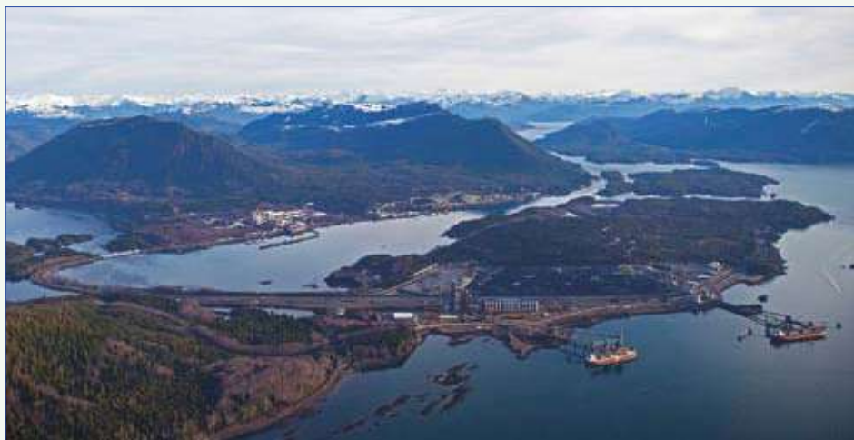
Construction of a $90 million Road, Rail and Utility Corridor to Ridley Island at the Port of Prince Rupert will support billions in new terminal developments and boost exports to Asia.
