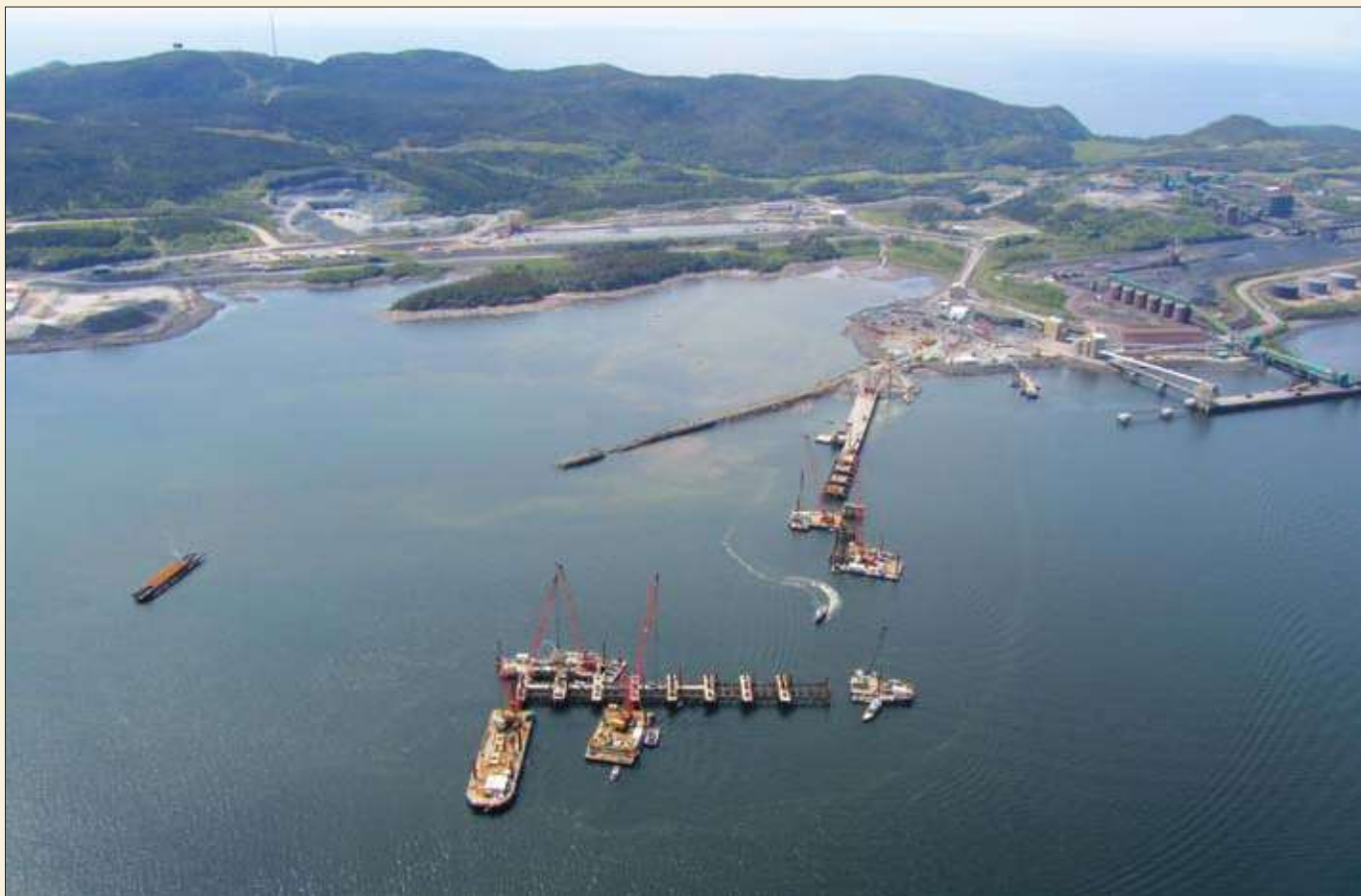
Construction of the new multi-user dock at Pointe-Noire in the Port of Sept-Îles is progressing well.
