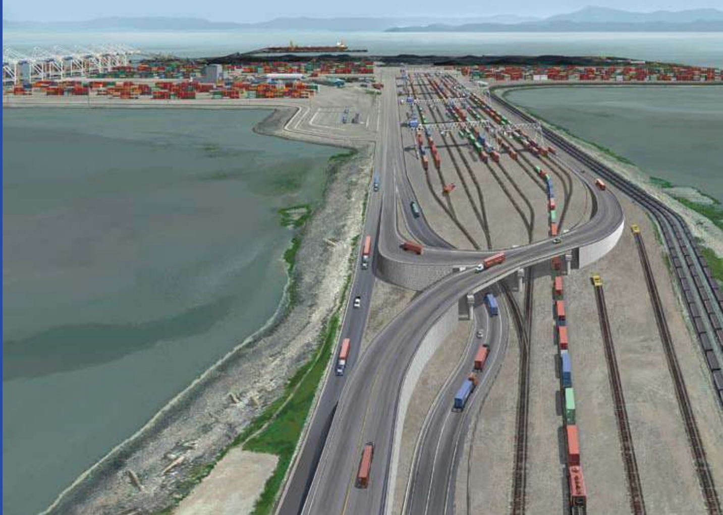
An overpass on the existing Roberts Bank causeway will separate road and rail traffic at Deltaport, Canada's biggest container terminal complex. Construction is slated for completion in late 2014.
