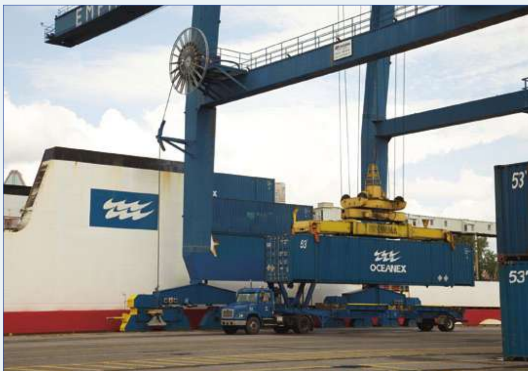
Oceanex ro/ro containerships call frequently at the Bickerdike terminal.
