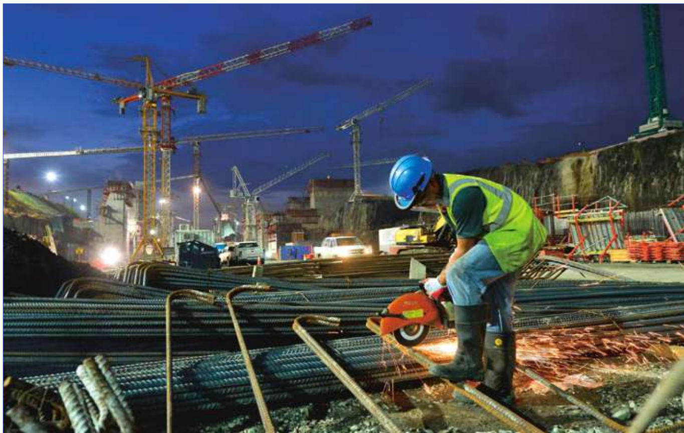
Panama Canal Authority
