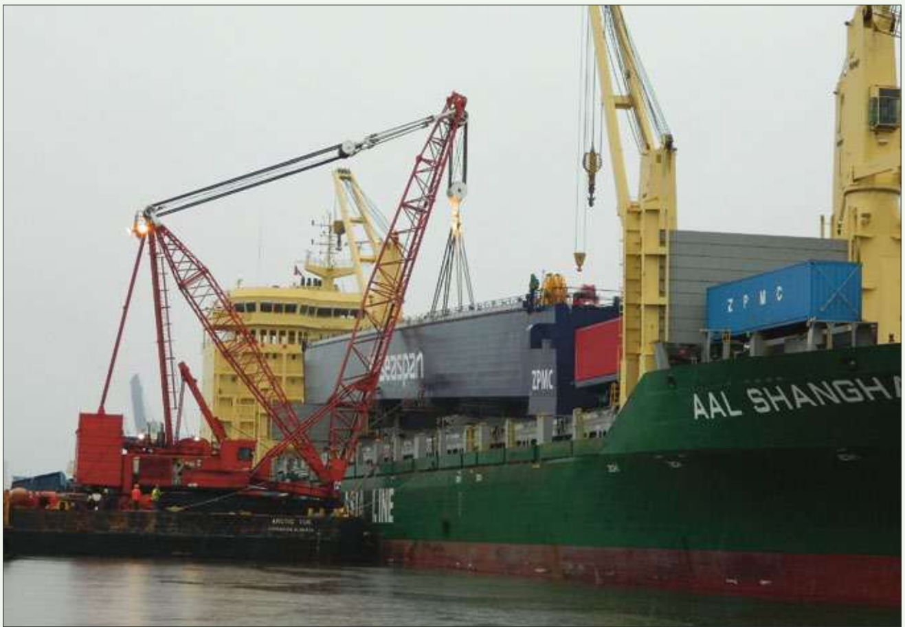
Heavy lift move involving equipment for Seaspans 300-tonne gantry crane, largest in Canada, at Vancouver Shipyards.
