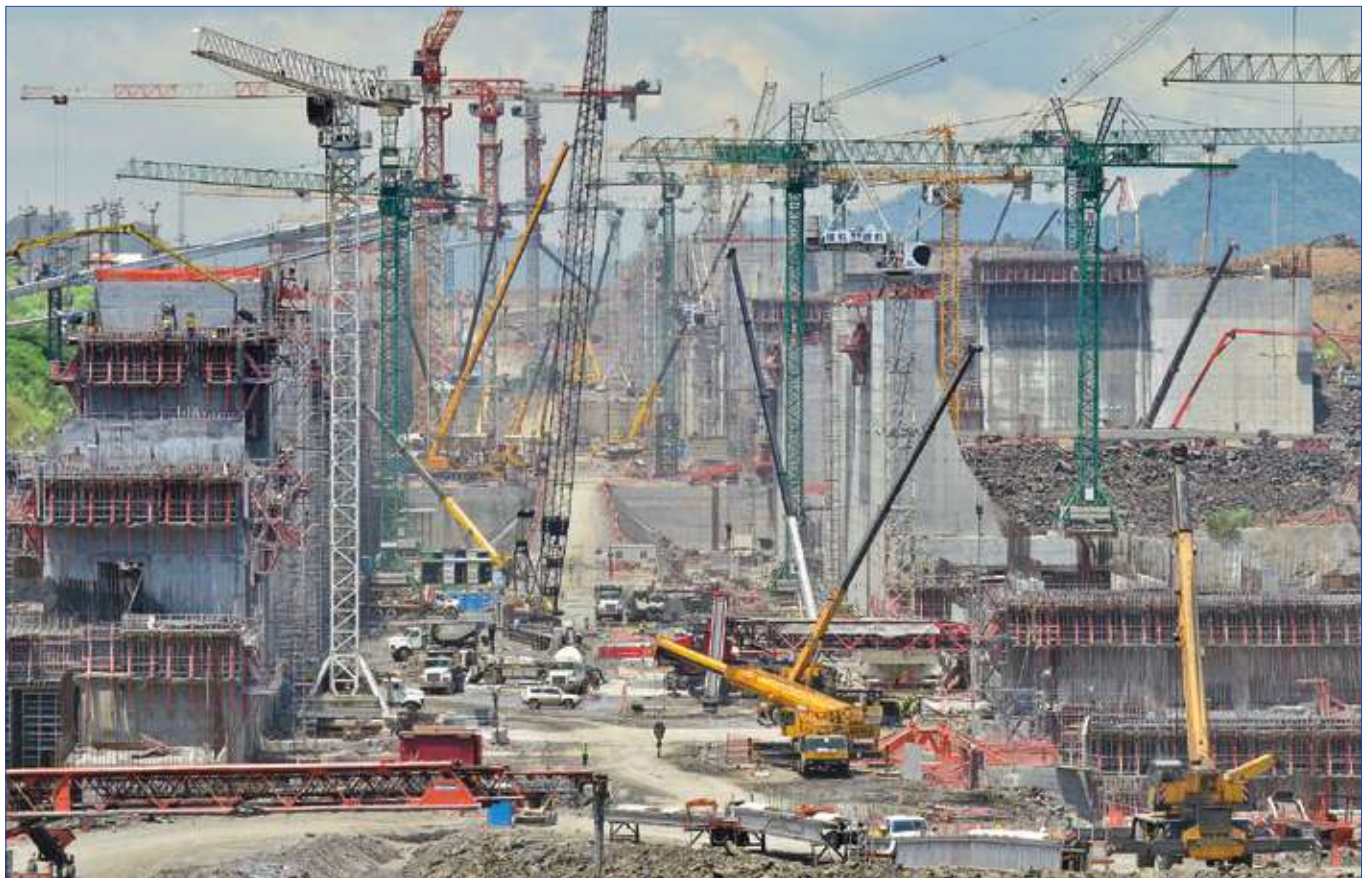
Panama Canal Authority
