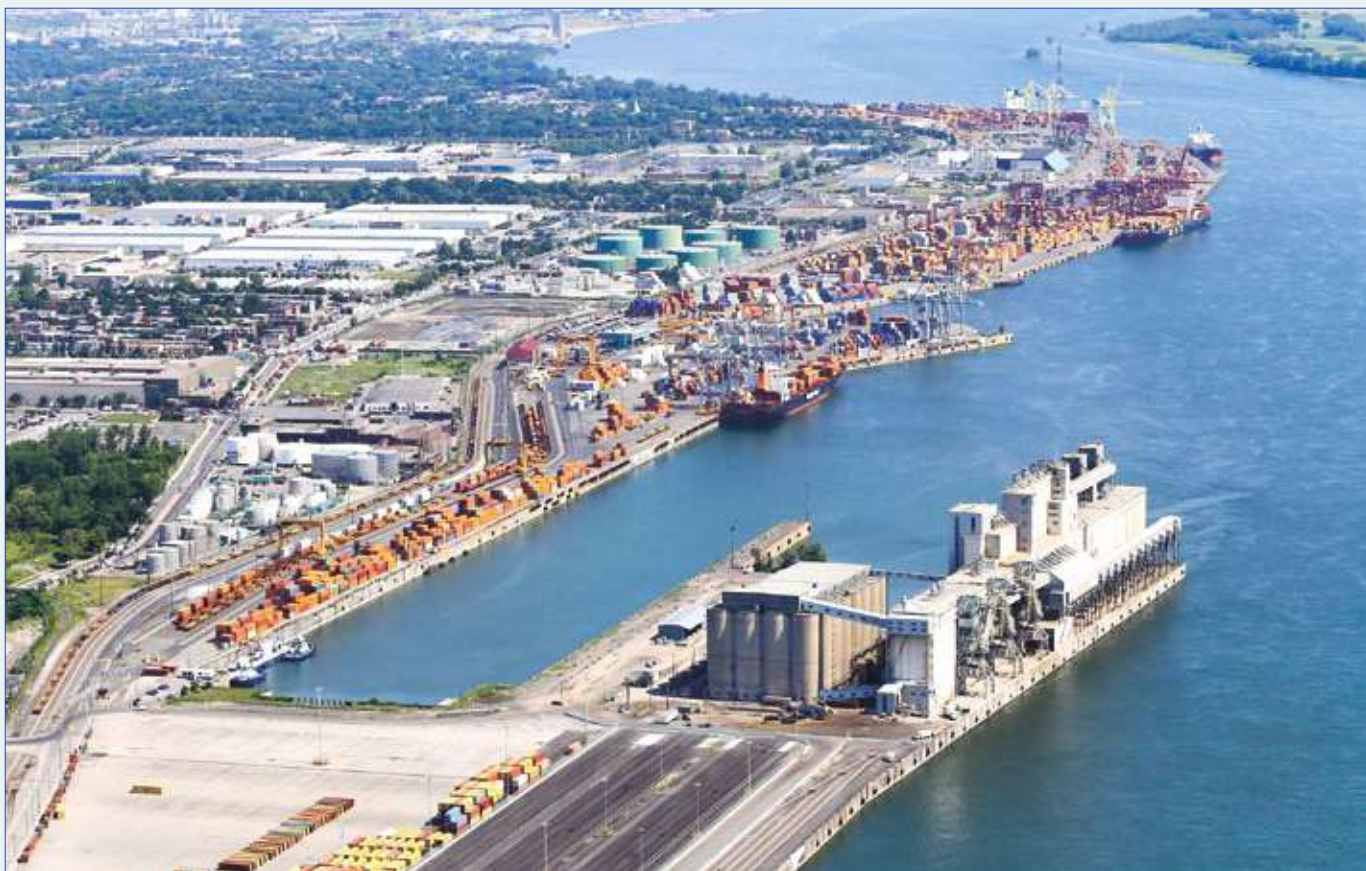
Deep in the hinterland of North America, the Port of Montreal is Canada's second biggest container port, capturing business from the U.S. Midwest and Northeast as well as from shippers in Central Canada.
