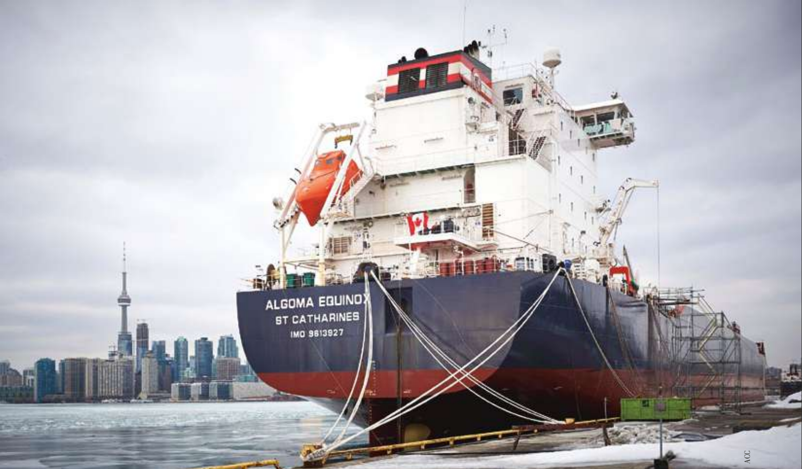
Algoma Central Corporation's new Equinox class ships have fully integrated exhaust gas scrubbers.
