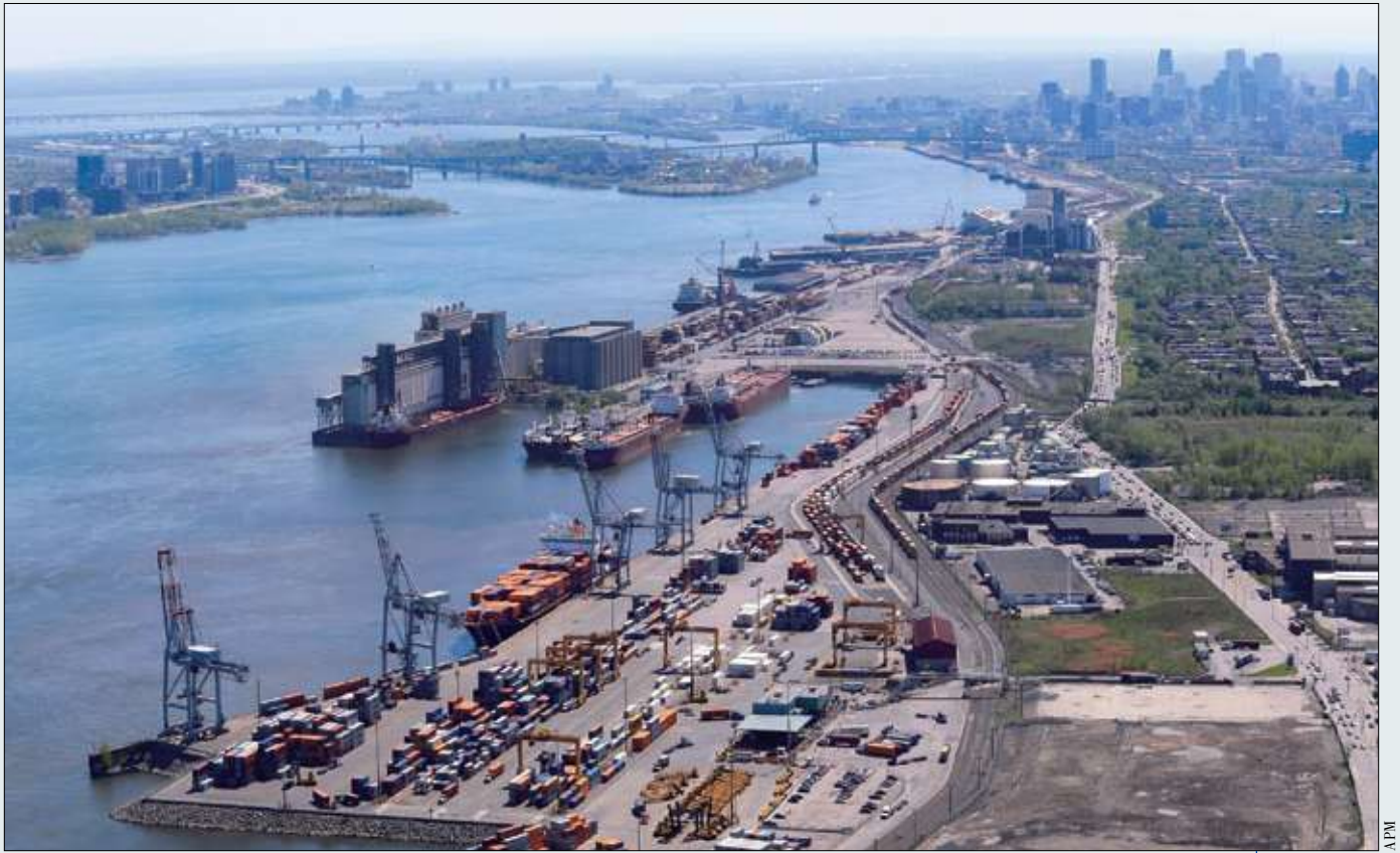
Aerial view of the Port of Montreal, Canada's leading gateway for North Atlantic trade.
