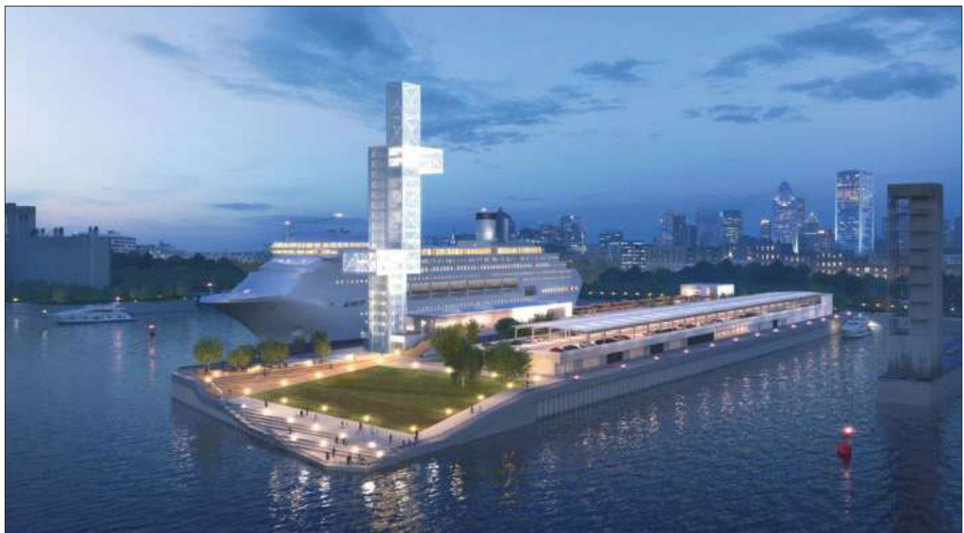
Artist rendering of new cruise facilities and observation tower under construction.
