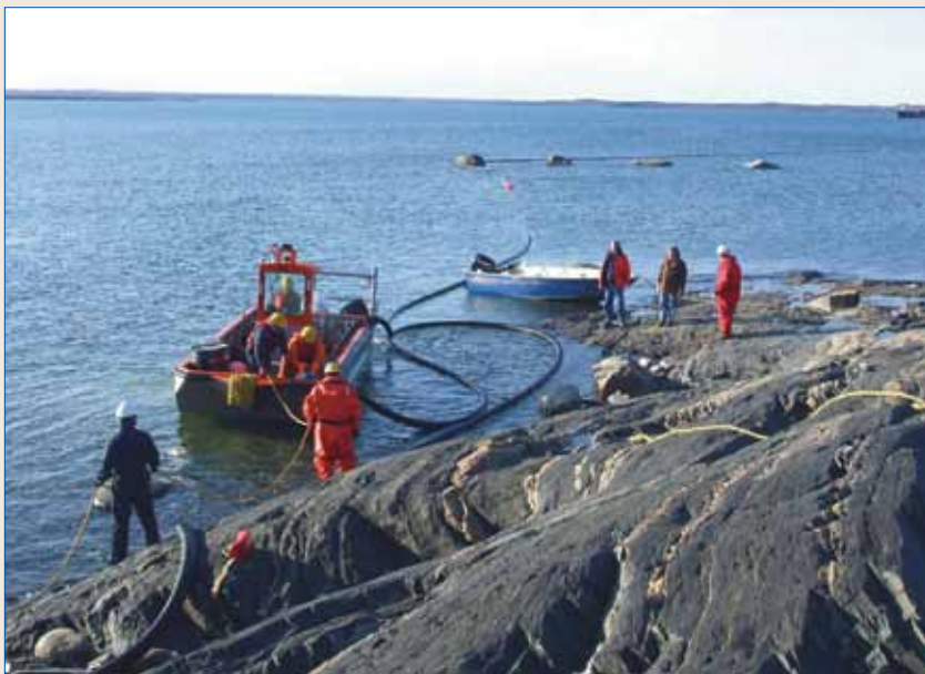
Crew bring hose to shore for a manifold connection.
