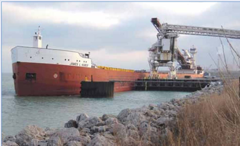
Port of Indiana-Burns Harbor
