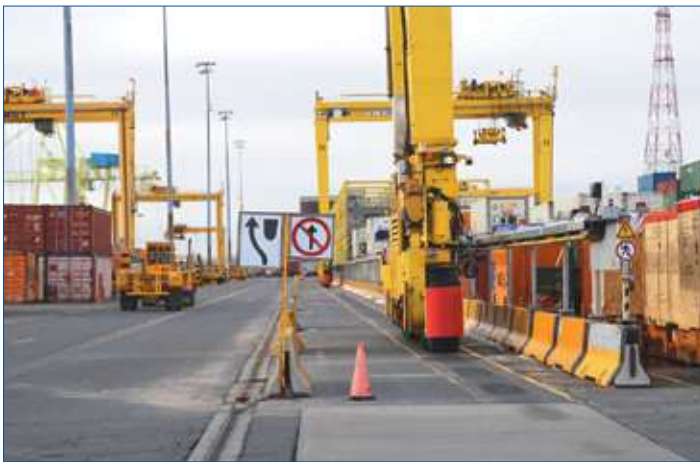
First Canadian container terminal to convert rubber-tired gantry cranes from diesel to electric power.
