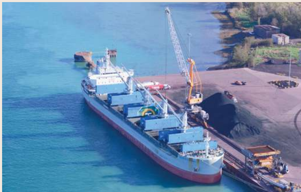
Aerial view of Logistec's bulk operations at the Contrecoeur terminal near Montreal on the St. Lawrence River.
