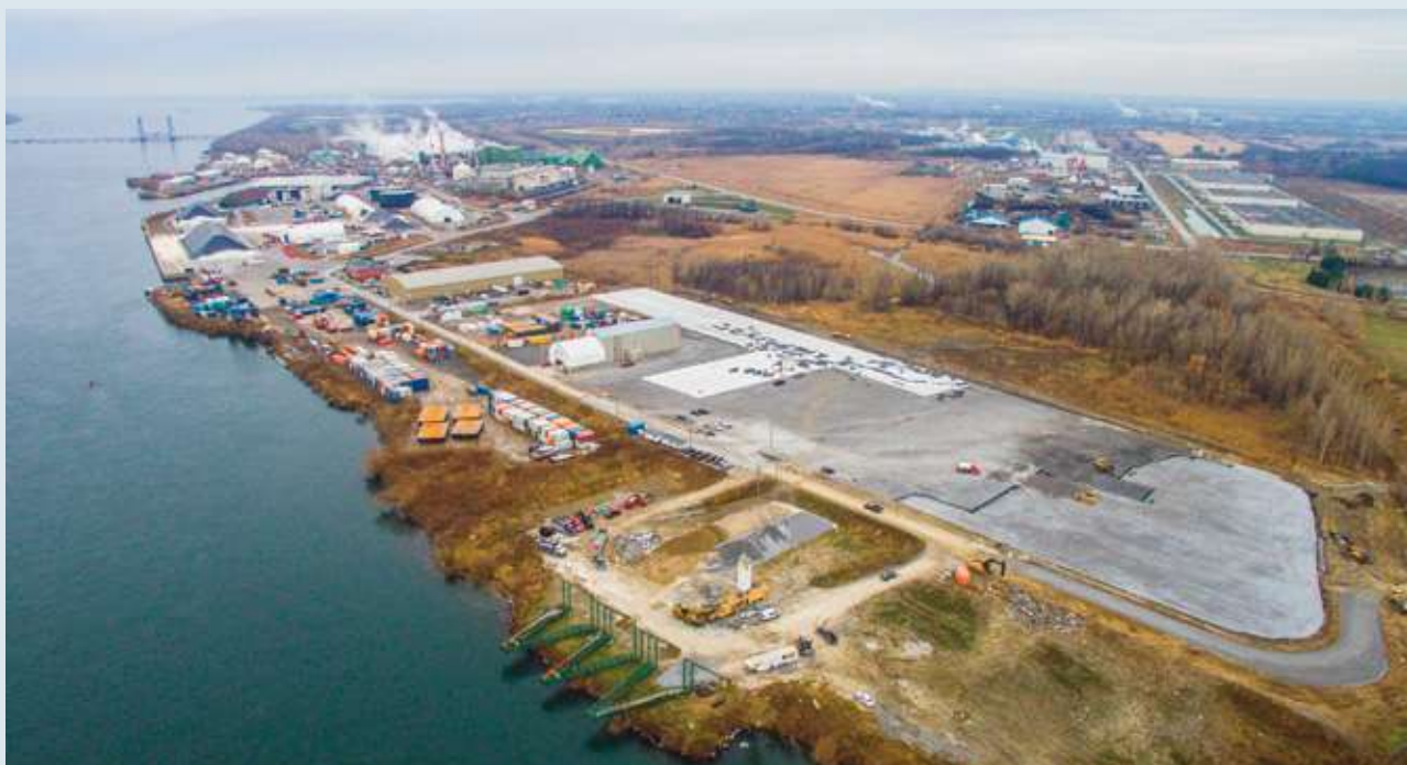
The Port of Valleyfield's new large laydown area will soon be ready to welcome breakbulk and project cargo.
