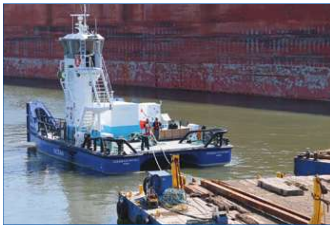
The Ocean Catatug in action pulling construction barges to the site of the new Champlain bridge.
