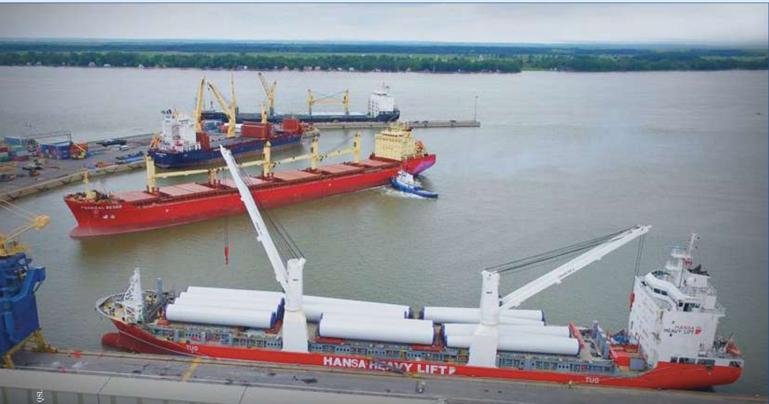
The QSL terminal at Bécancour offers versatile outdoor and indoor storage facilities to receive dry bulk, steel, breakbulk and project cargoes.
