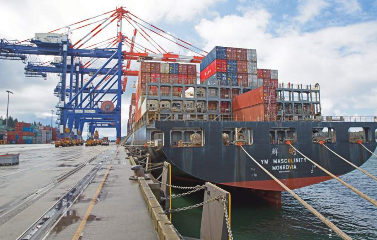
Next expansion phase will boost the capacity of Prince Rupert Container Terminal to 1.8 million TEUs by 2022.
