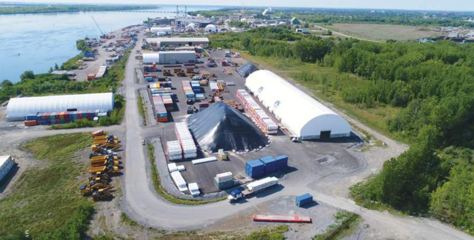
The Port of Valleyfield's enlarged laydown area is spiking new business opportunities.
